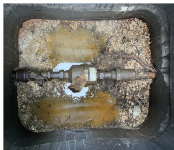
A meter box contaminated with waste oil.
