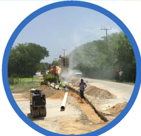
Work continues in the Brac.
