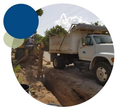
Works to upgrade the 6-inch pipeline, to 8-inch pipes, on Cross Road, between the West End Water Works and the intersection with the West End Road was scheduled to begin in April. However, the project was delayed by several weeks due to equipment issues with the trencher. Vermeer Once repair works were completed, work resumed on the project in June and was completed in November. Work
