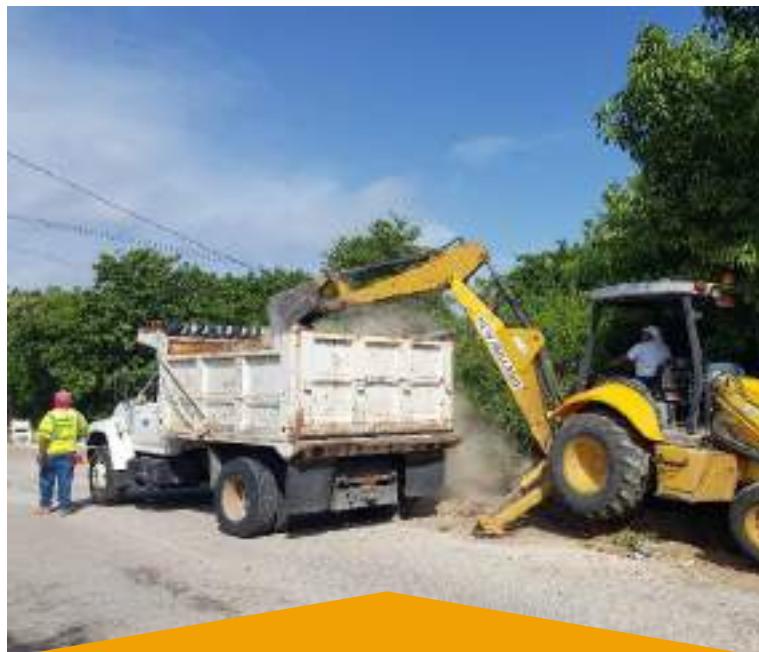
Work continues in Cayman Brac to expand the piped water network and remediate sections of existing pipeline to ensure operational efficiency.
