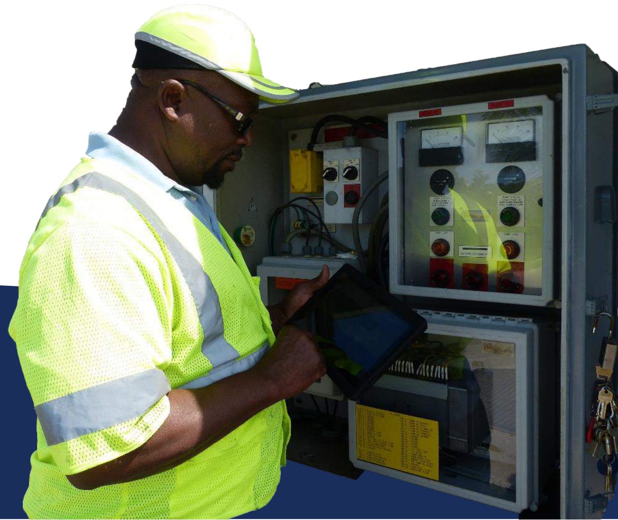
The wastewater team conducts daily readings of wastewater pump houses, to monitor the function of the system.
