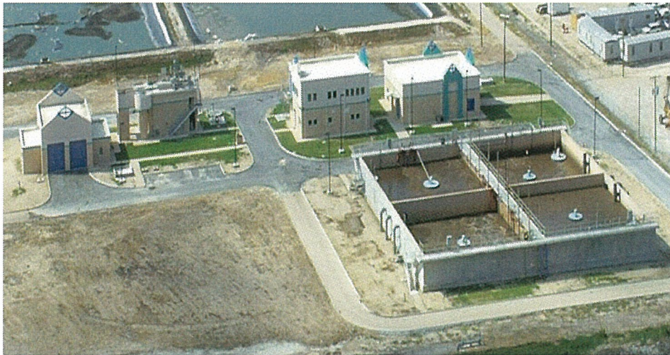
New Grand Cayman Wastewater Treatment Works April 2005
