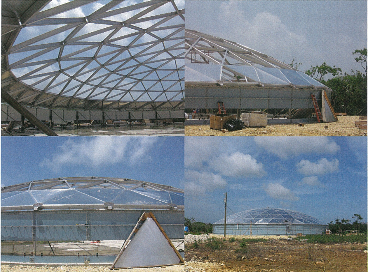
Construction of North Side Reservoir June 2006
