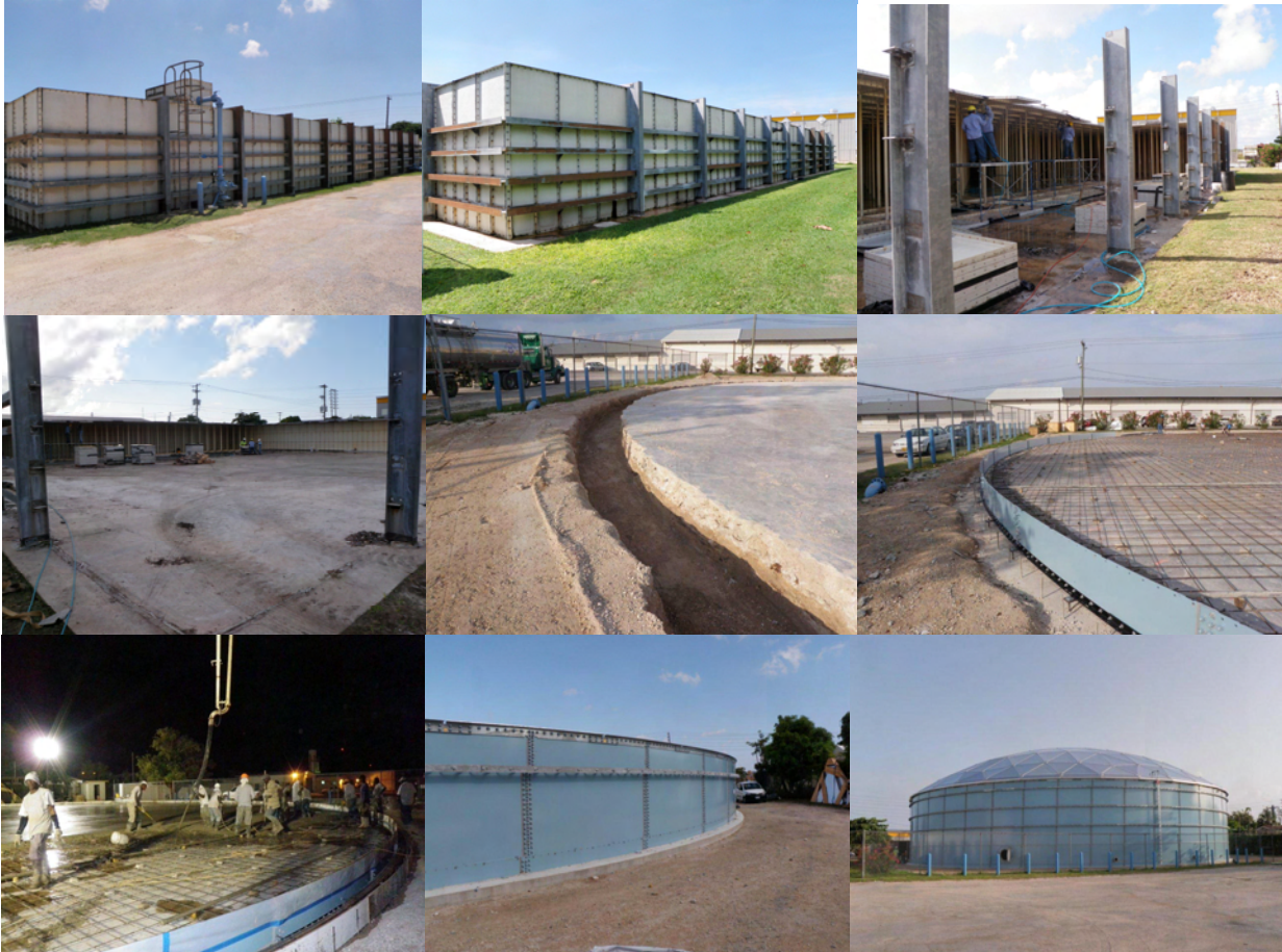
Water Authority Red Gate Reservoir #1 Demolition & New Tank Erection – October 2011 to June 2012
