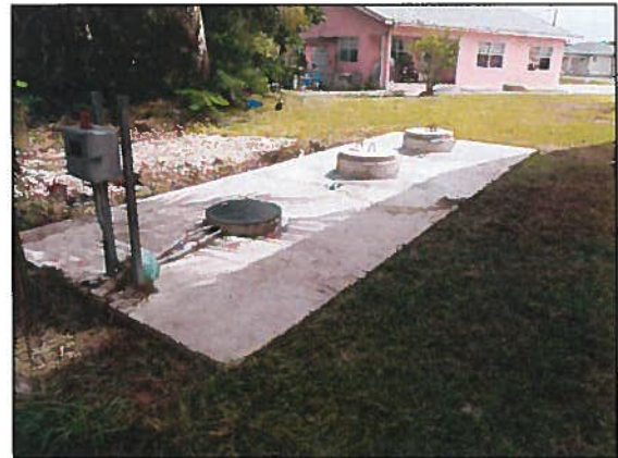
Randyke Gardens Wastewater Plant Upgrade
