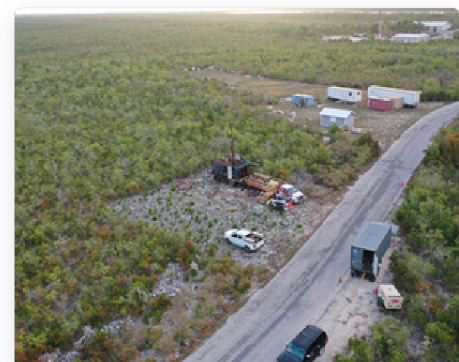
Image: The pilot well drilling took place at the future site of the Bluff Water Works in Cayman Brac
