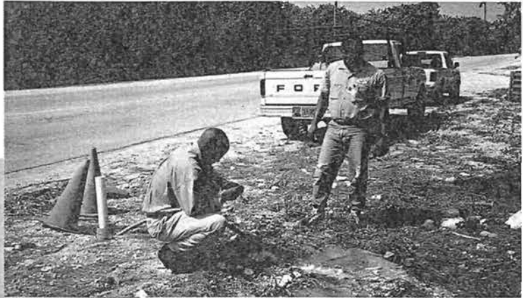
Civil Engineer, Troy Whittaker and Superintendent-NW, Jack Hunter check chlorine residuals after disinfecting new water mains
