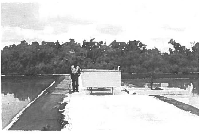
Experimental work being carried out on the sludge accumulation in the sewage treatment works
