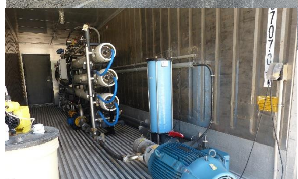
The Authority's containerised RO plant will one day be transferred to Little Cayman.
