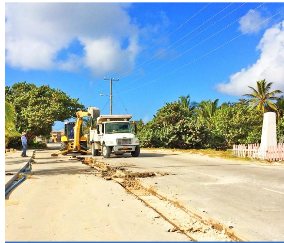
Work on the Bodden Town Pipeline Project progressed steadily in 2016.
