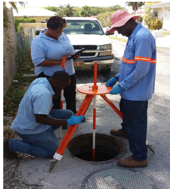
Members of the Wastewater team use a GoPro mounted to a specialty rig designed in-house to survey manholes safely and efficiently.
