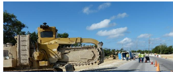
Work on the Linford Pierson Highway as part of the road expansion began in 2016.
